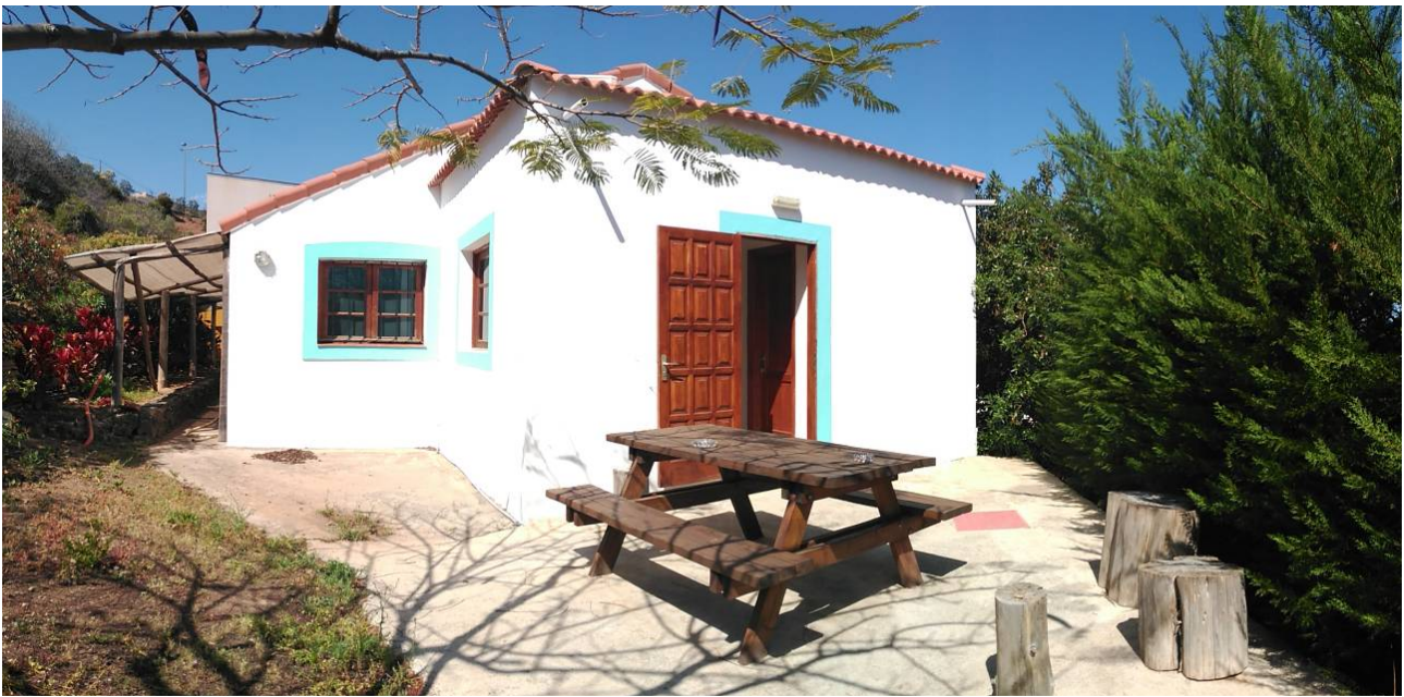
Vista general exterior Trasera / Office
