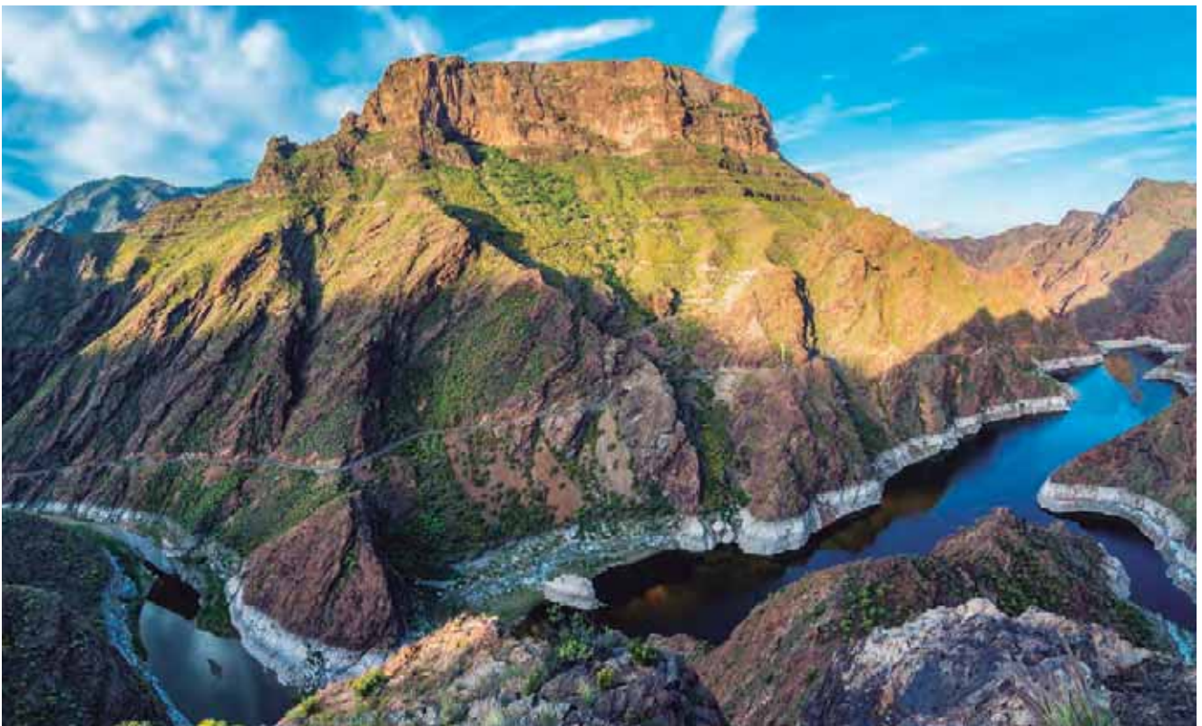
Figure 2. a.176. View of El Parralillo dam at the foot of La Mesa del Junquillo. The dam collects the waters from El Carrizal Ravine, Merino Ravine and Tejeda Ravine, known as La Aldea Ravine further downstream. It is managed by the Comunidad de Regantes de La Aldea (La Aldea Water Rights Community), an area outside and to the west of the area of the proposed property. © Orlando Torres
