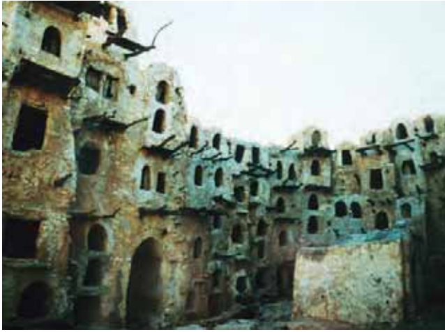
Figure 2.a.44. Qsar Nalut fortified collective granary in Djebel Nefusa, Libya. © Juan Antonio Belmonte
