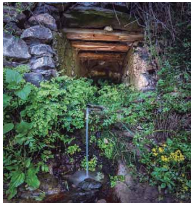
Figure 3.2.37. Small water mine with filtering gallery in El Hornillo © FEDAC
