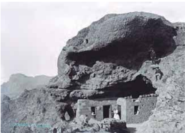
Figure 2.a.94. Cave dwelling in the middle of the last century. La Cilla, Artenara. Source; Ayuntamiento de Artenara
